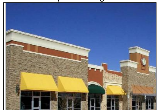
Fig. 24 Window trims and awnings add to the visual character of the fenestration.
