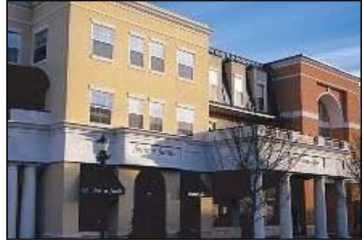
Fig. 18 Bays & entryways break up this façade.
