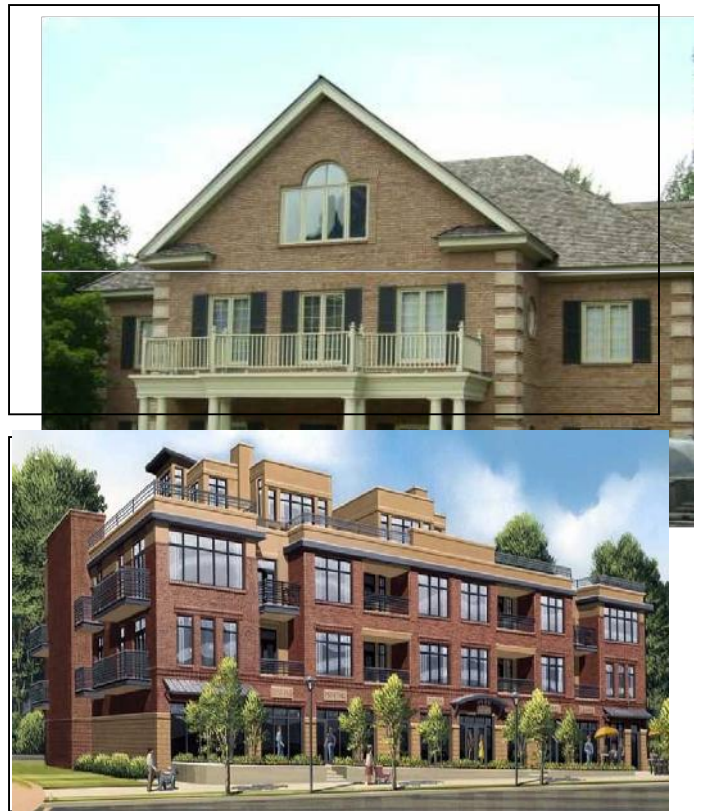
Fig 1. Brick is a classic and timeless building material.
