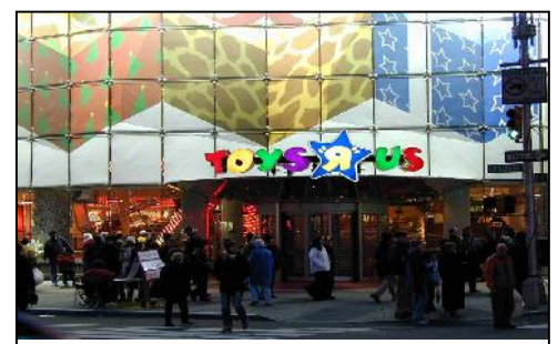
Fig. 10 Bright colored signs that distract from the façade are not desirable.
